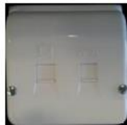
FTTC: Dual Interface Copper Pair NTU – Master Socket
